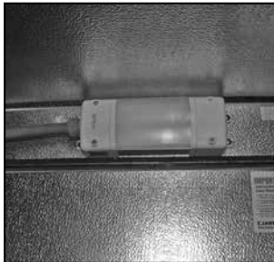
ABOVE DOOR LED LIGHT FIXTURE
