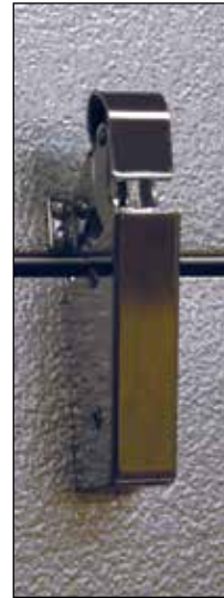
Spring actuated door closer
